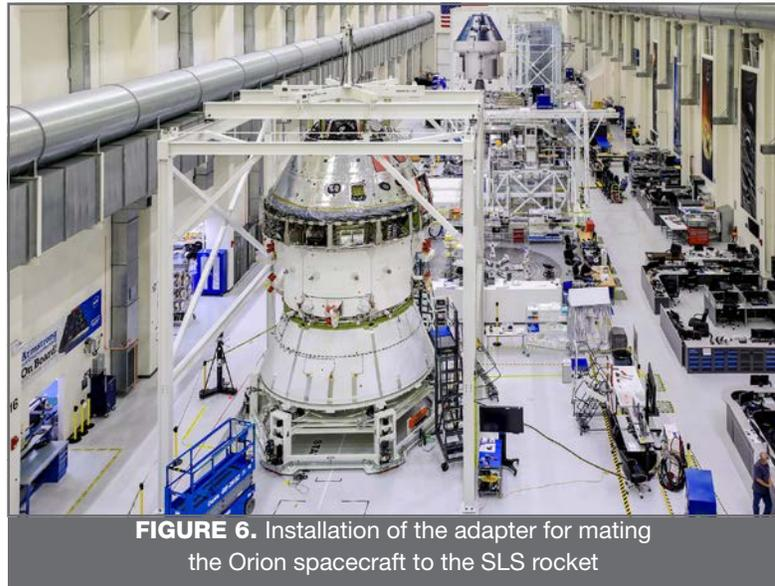
**FIGURE 6.** Installation of the adapter for mating the Orion spacecraft to the SLS rocket
