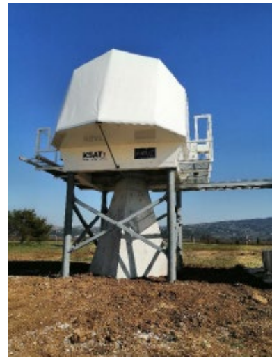
Figure 11.35: KSAT's low-complexity optical ground station in Nemea (2021).
