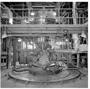
Image 191: Kiwi-B engine inside the B-1 Stand (GRC-1964-P-01347).
