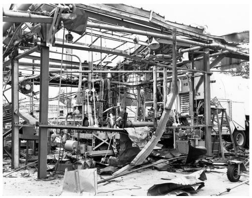
Image 92: Damage to the Pilot Plant's Pump Building following a hydrogen explosion in September 1964. The test rig is visible near the center of the structure, and a liquid-hydrogen trailer is to the right (GRC-1964-P-01562).
