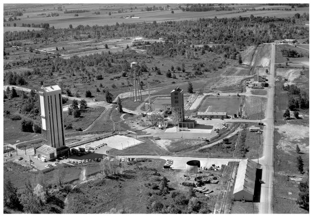
Image 104: The B Complex included the Pump and Shop Building, a substation, two boiler buildings, a Valve House, and the steam ejector apparatus. The B Control Building is visible in the upper right corner (GRC–1964–C–72620).
