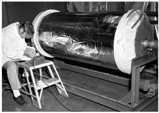
Image 145: A technician installs insulation on a calorimeter for testing in K Site (GRC-1971-P-01416).
