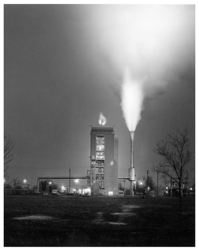
Image 1: Testing of a hydrogen flow system for a nuclear engine in the High Energy Rocket Engine Research Facility (B–1 Stand) in June 1965 (GRC–1965–P–02327).
