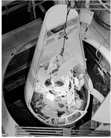
Image 128: Technicians install a mock-up Surveyor spacecraft atop the Atlas/Centaur in the E Stand (GRC–1964–P–01239).
