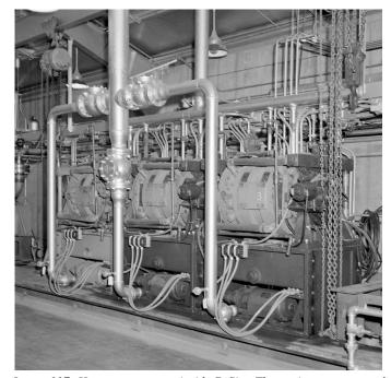
Image 117: Hot gas generator inside D Site. The equipment was used to supply gaseous hydrogen to experimental turbines to simulate the first stage in nuclear engine startups (GRC-1961-C-55372).
