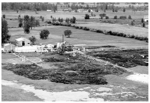
Image 93: Damage at the Pilot Plant following a liquid-hydrogen explosion on 14 September 1964. The blast convinced engineers to install a protective concrete wall inside the H Control entrance (GRC-1964–P-1559).
