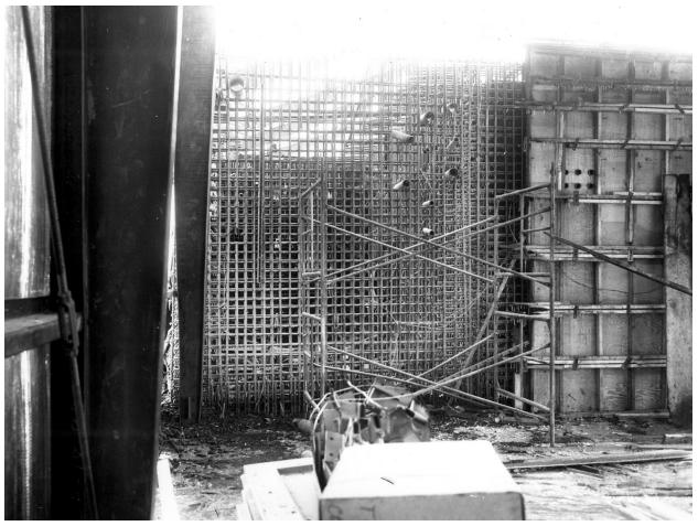
Image 46: Construction of F Site in December 1958. Electrical and hydraulic flow problems delayed testing until July 1963 (GRC–2016–C–07418).
