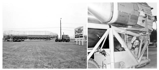
Image 79: Atlas missile is delivered to Plum Brook in July 1963. The Image 80: General Dynamics designed a unique 64-footvehicle had to avoid tight turns, most bridges and underpasses, and large urban areas during its 2,500-mile trek from the General Dynamics plant in San Diego to Sandusky. (GRC-1963-C-65589).
