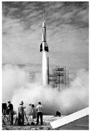
Image 13: Launch of a V–2/WAC (Without Any Control) Corporal rocket in 1950 (NASA 66P–0631).
