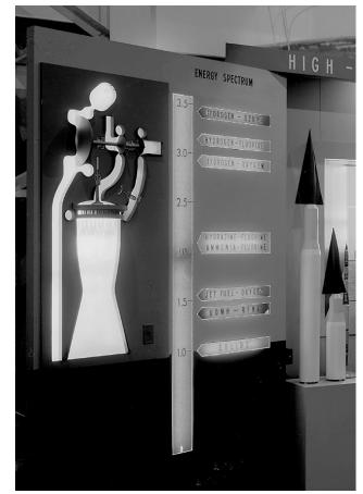
Image 31: Display at the RETF stop during the NACA's 1957 Inspection. The panel compares the performance of several rocket propellants, including hydrogen-oxygen, hydrogen-fluorine, kerosene, hydrazine, and solid fuels (GRC–1957–C–46150).
