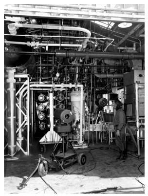
Image 96: Fluorine pump rig inside I Site. Two cameras are set up to film the test (GRC–1962–C–59411).
