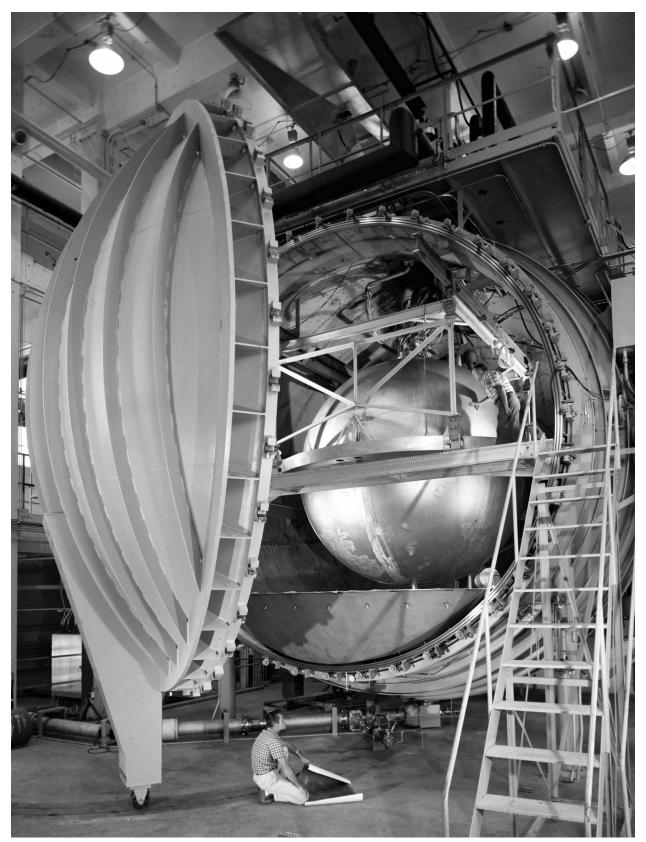
Image 129: A 13-foot-diameter propellant tank installed inside the Cryogenic Propellant Tank Facility (K Site) vacuum chamber (GRC-1967-C-03315).
