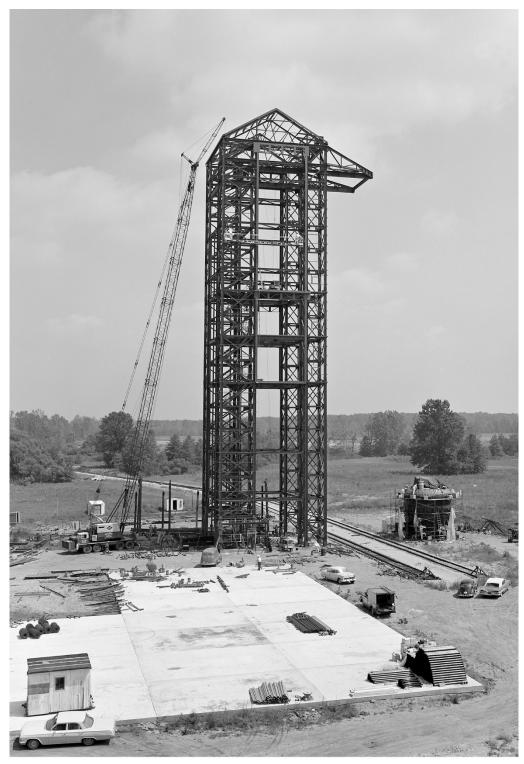
Image 103: Construction of the B–3 Stand began in the spring of  $1963.^{445}$  Construction crews assembled the steel framework during the summer and added the siding and platforms in October. The basic structure was complete by mid-November 1963. The next year and a half were spent installing the other infrastructure and support systems, including the connection to the B–1 altitude exhaust system (GRC–1963–P–01751).
