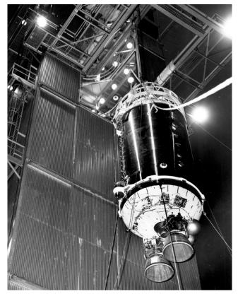
Image 75: A Centaur stage is lifted into E Stand just before dawn in January 1964. Centaur was powered by two Pratt & Whitney RL–10 engines, which ran on liquid hydrogen and liquid oxygen (GRC–1964–P–01084).
