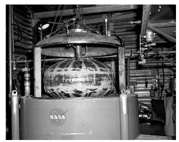
Image 89: Linde superinsulated tank at the J–3 facility in May 1963. The 150-gallon stainless steel tank was designed to be suspended by its neck, so it was not a true space tank (GRC–1963–P–01446).
