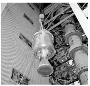
Image 192: Kiwi-B reactor is lifted into the B–1 Stand (GRC–1963–P–01358)
