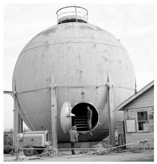
Image 231: J-5 containment vessel (GRC-1960-C-54830).
