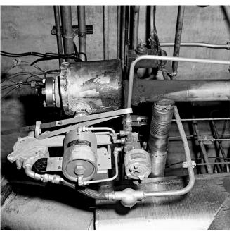
Image 203: A 60,000-rpm turbine at D Site (GRC-1962-C-59323.
