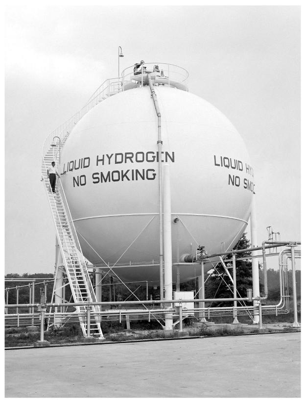
Image 6: A 200,000-gallon hydrogen Dewar, the largest in the world at the time, at Plum Brook's B Complex (GRC–1965– P–02438).
