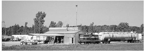
Image 62: Gas Handling Area with both a railcar Dewar and roadable Dewars. The site was located just north of E Stand (GRC-2016-C-05788).
