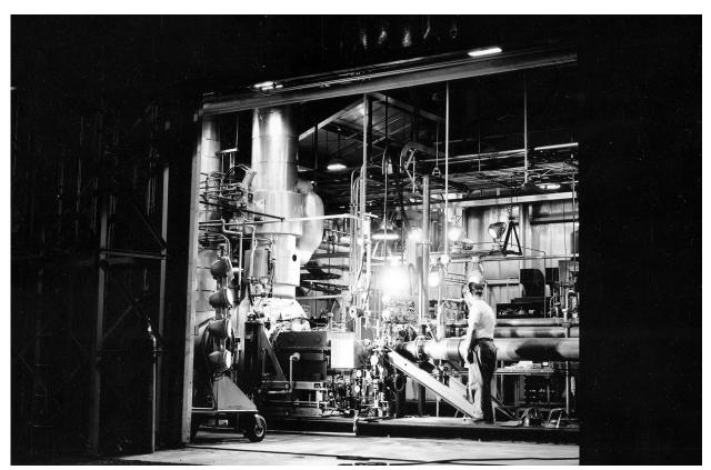
Image 112: View into the Liquid Hydrogen Pump Facility (A Site). Lewis researchers used the hydrogen loop extensively in the 1960s to study centrifugal and multistage axial-flow pump configurations (GRC–1963–P–01196).
