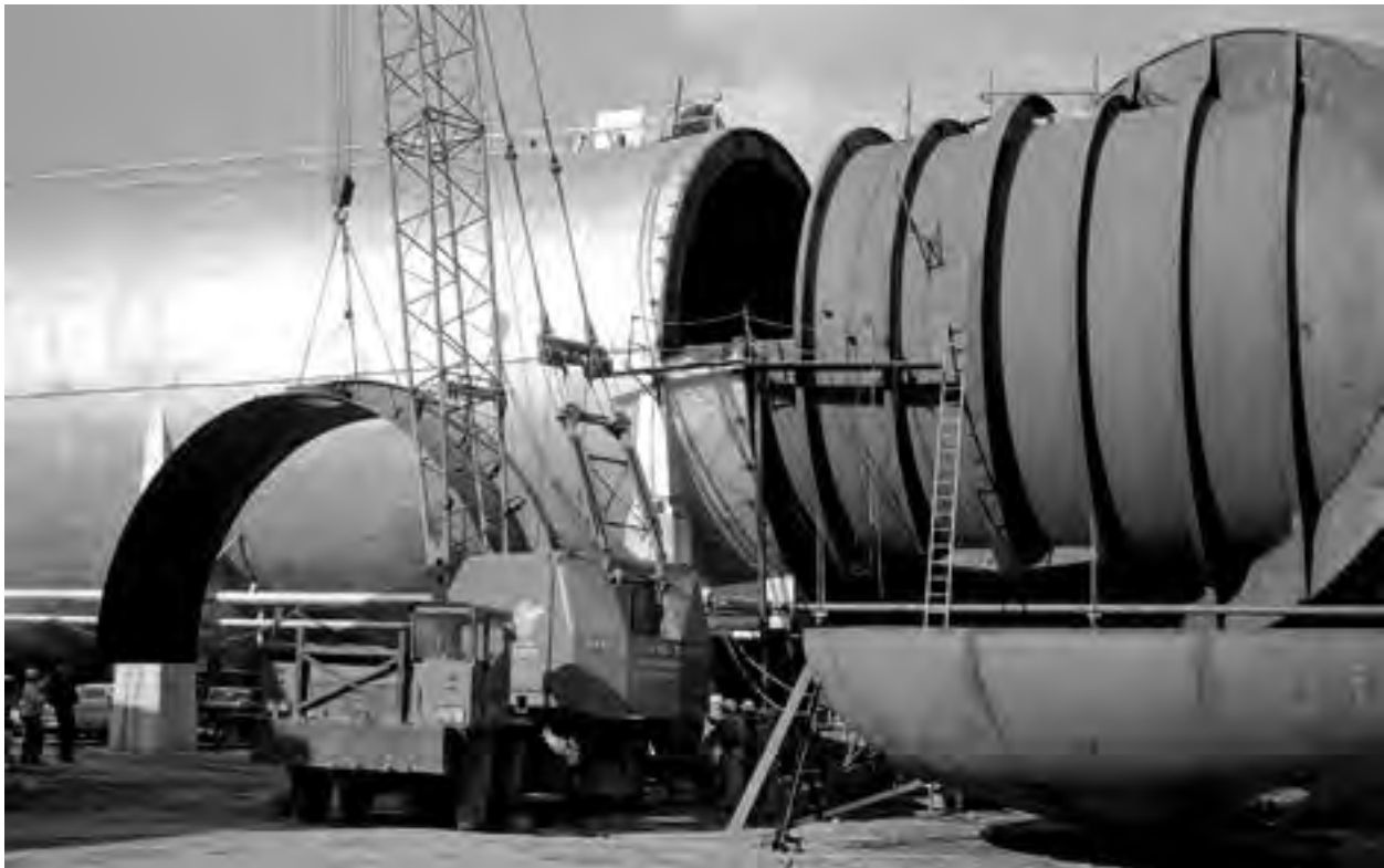
Image 191: Three bulkheads were placed inside the AWT to create the SPC. The largest is seen here being inserted approximately where the wind tunnel fan was located (NASA C-1961-58551).
