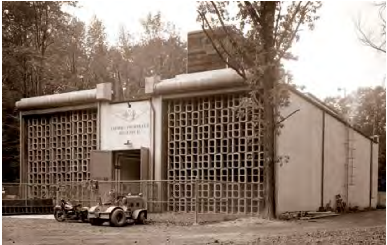
Image 34. In May 1942 the Prop House became the first operating facility at the AERL. It contained four test cells designed to study large reciprocating engines. Researchers tested the performance of fuels, turbochargers, water-injection, and cooling systems here during World War II. The facility was also used to investigate a captured German V-I buzz bomb during the war (GRC-1942-C-01134).
