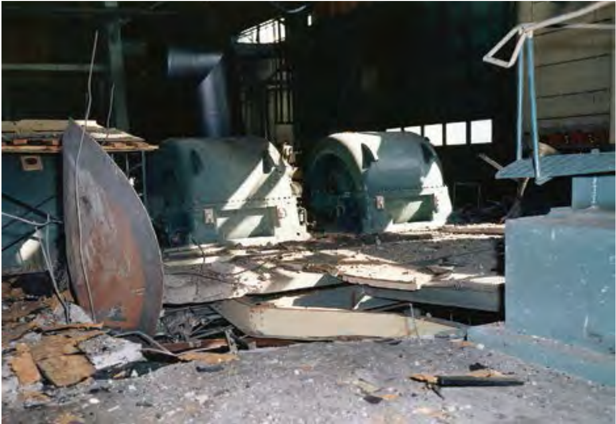
Image 241: Damage to the PSL Equipment Building (GRC-1971-C-01422).
