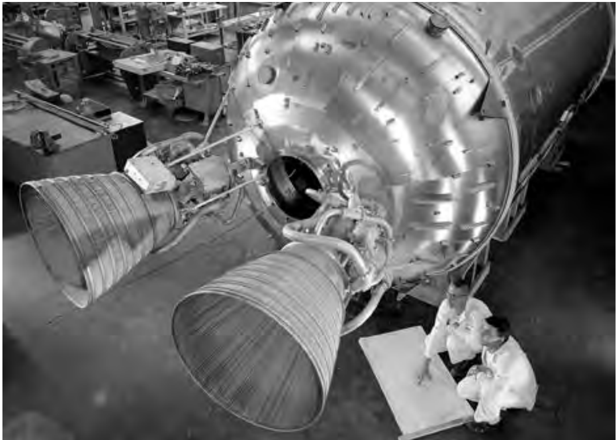
Image 165: Lewis technicians examine a Centaur rocket in the Space Power Chambers shop (GRC–1964–C–71100).
