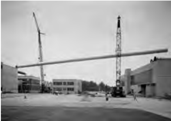
Image 144: The overhead air-handling line between the PSL and the 8×6 is installed in 1954 (GRC-2007-C-025662).
