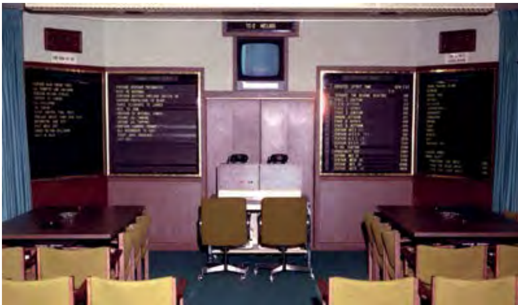
Image 277: Centaur rocket control room in the Development Engineering Building during the preparations for the Titan-Centaur-Helios launch on 10 December 1974. From here the Lewis staff in Cleveland could monitor and back up the Lewis launch team in the actual control room at Cape Canaveral (GRC-1974-C-04007).
