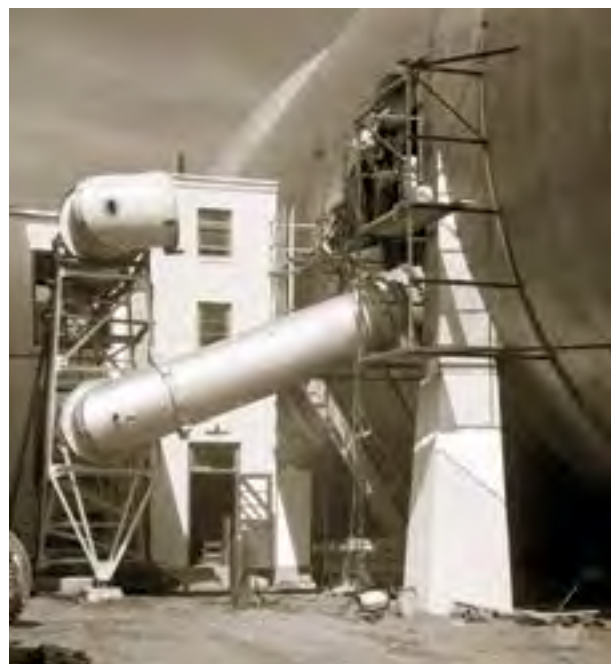
Image 112: Construction of the lab's first supersonic tunnel. Eventually the building would house three small supersonic tunnels (GRC-1945-C-10764).
