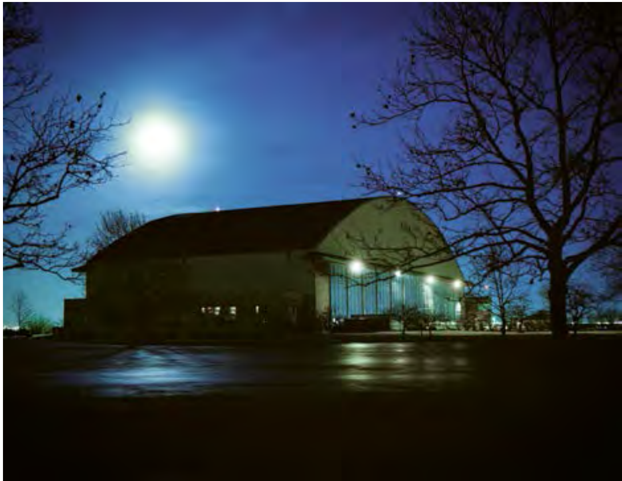
Image 289: The Lewis hangar in November 1981 (GRC-1981-C-05731).
