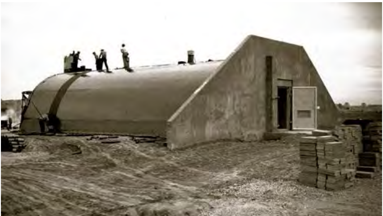
Image 29: Construction of one of the 99 concrete bunkers used to store explosives, c1941 (GRC-2015-C-06817).
