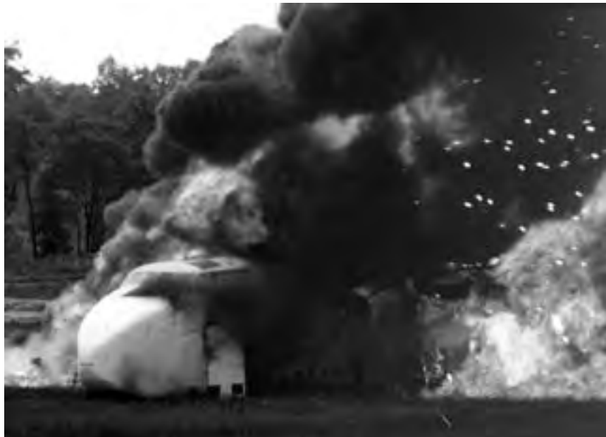
Image 139: Lewis researchers crash a transport aircraft through barriers at the Ravenna Arsenal. Incandescent particles are visible from the explosion (GRC-1957-C-43929).
