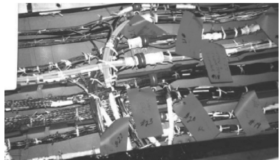
Figure 21 -- OV103 Mid-Body: Intersecting Wire Bundles
