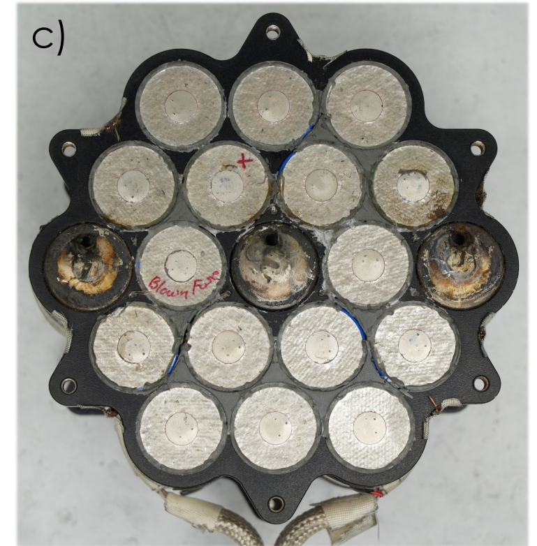
Figure: following the removal of bussing material for inspection of heat sink between cells.
