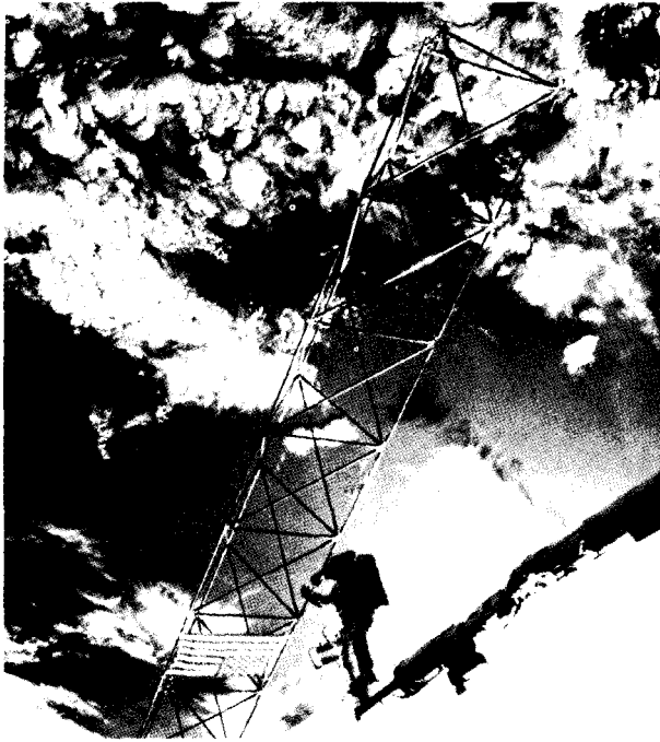
On the last flight of 1985, STS 61-B, Astronauts Jerry L. Ross and Sherwood C. Spring demonstrate the ease with which large structures can be assembled in space.
