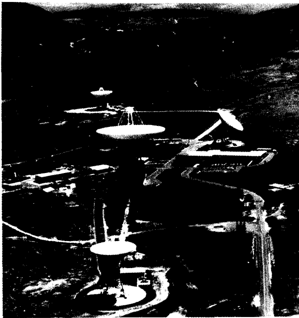
Consolidated Ground Network facilities, Canberra, Australia.
