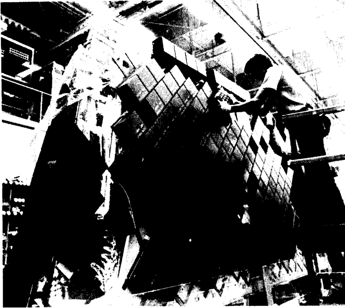
Therm-O-Trol, a metal-bonded foam insulation derived from space research, is applied along the 1300-kilometer-long Alaskan oil pipeline to retain the 82°C temperature at which crude oil will continue to flow.
