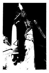
having flown the approach and landing test flights in 1977, was airlifted to the Marshall Space Flight Center. In May 1978 it was hoisted (lower left) into the dynamic test stand and joined (lower right) to the external fuel tank and two solid-rocket boosters for vibration testing of the total Shuttle configuration.
