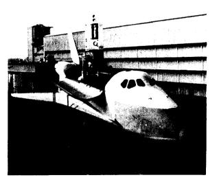
This mockup of the Space Shuttle orbiter was used to make detailed studies of a full-scale model of the Low Cost Modular Spacecraft. This spacecraft was one of several modular configurations being studied by NASA's Goddard Space Flight Center as economical means to place spacecraft into orbit from the orbiter and later to resupply or retrieve them. The first prototype orbiter is scheduled for rollout in September 1976.
