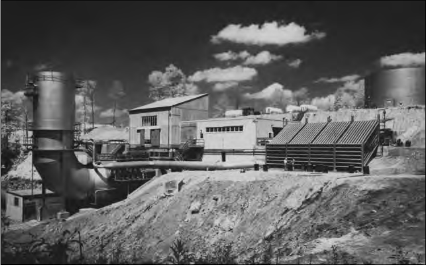
The $2.5 million Rocket Engine Test Facility (RETF), viewed from the Abram Creek valley shortly after construction, was completed in 1957. The RETF was an experimental facility, capable of testing sub-scale engines and components up to 20,000 pounds of thrust. NASA C-45652
