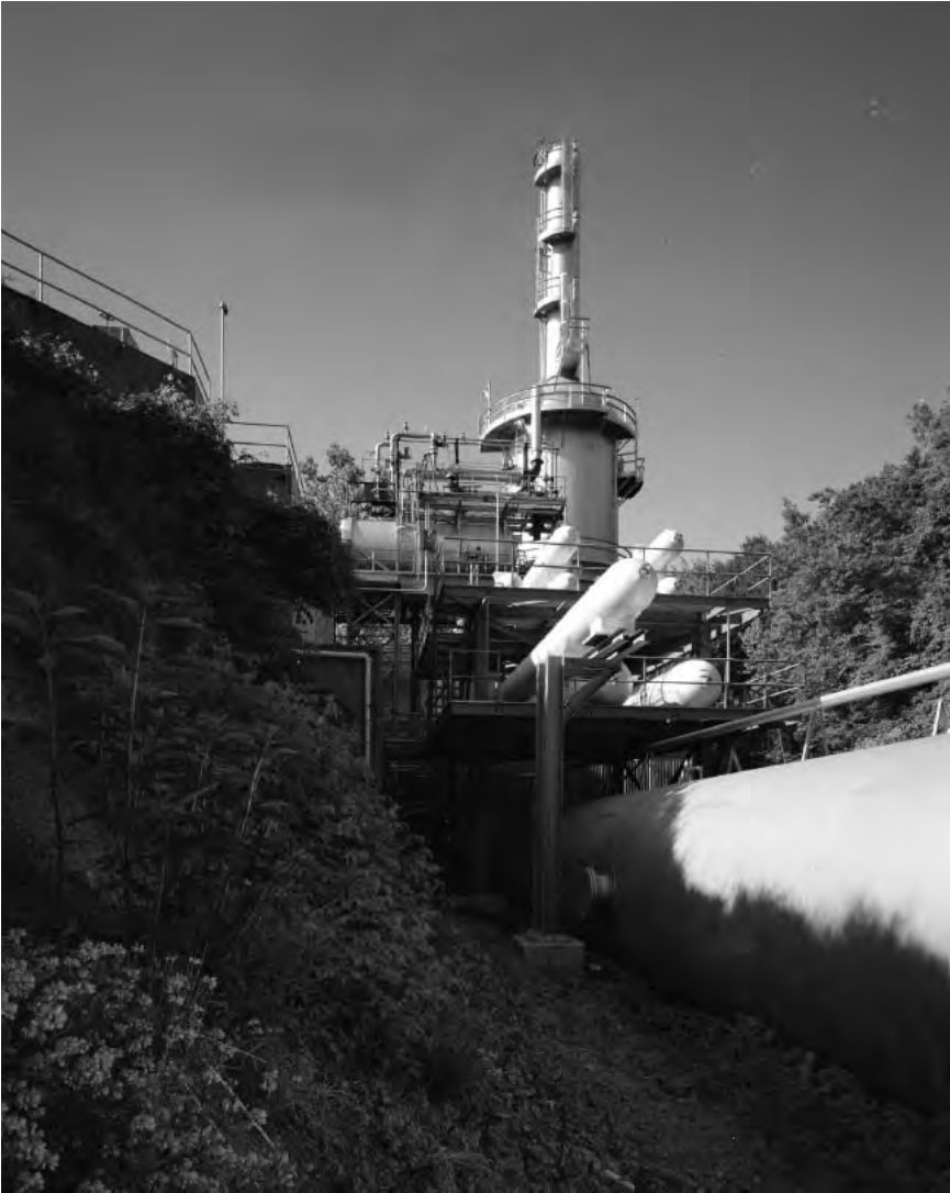
The RETF after the $1 million modification to create the new altitude facility (Stand B), 1985. This modification made the RETF even more versatile, allowing engineers to rapidly switch instrumentation and control from one test stand to the other.
