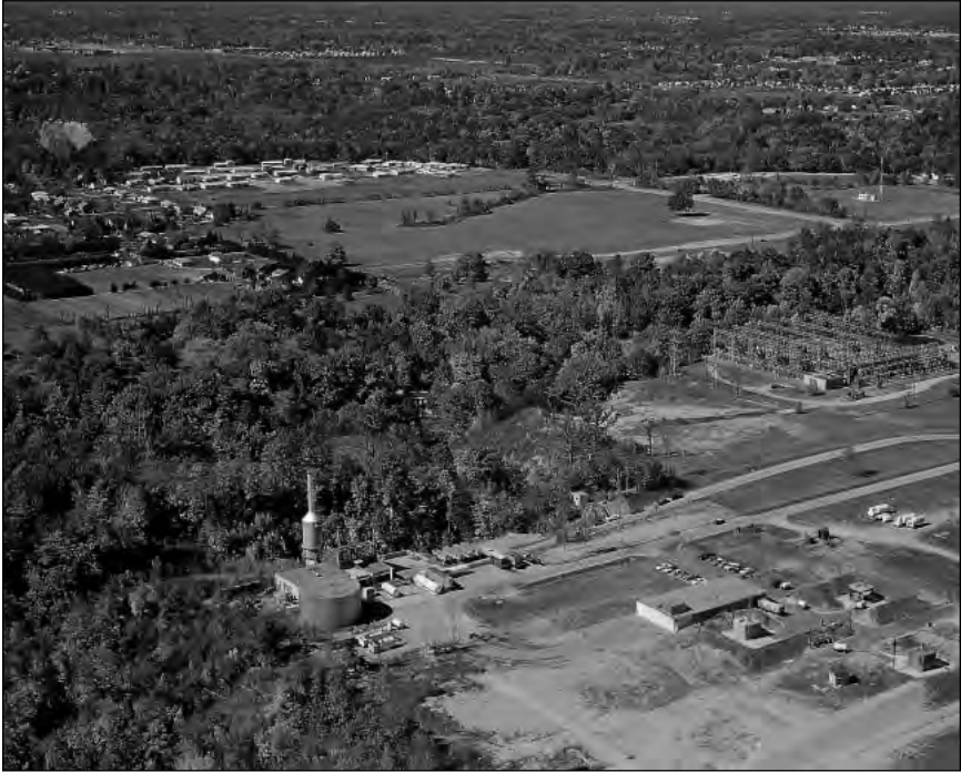
Aerial view of the RETF in 1963. The old rocket engine test cells can be seen (lower right), protected by earthen mounds. The woods separated the RETF from residential areas of Brook Park to the south.
