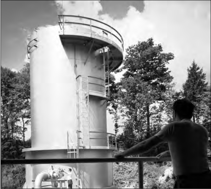
A technician looks from the test cell doorway toward the scrubber, 1957. NASA C-45734.
