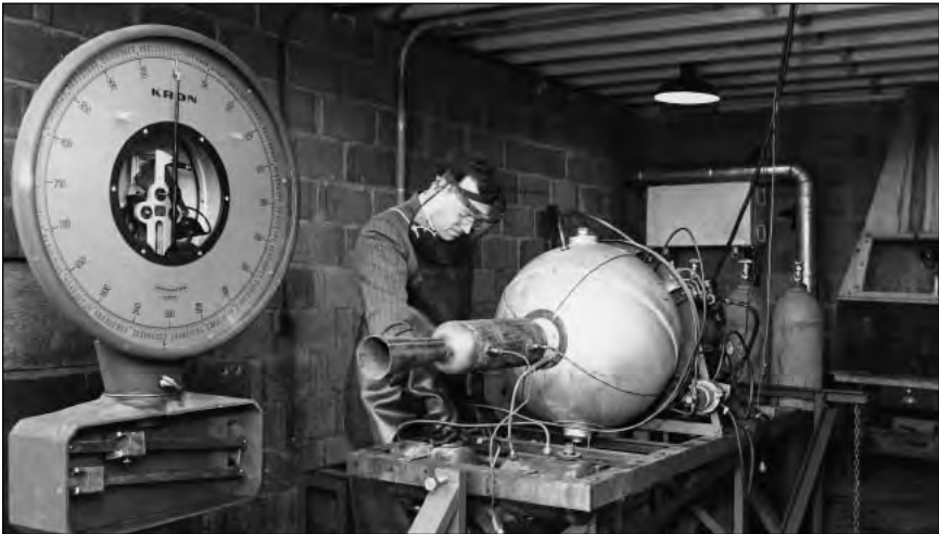
Preparing jet assisted take-off units, called JATOs, for testing in one of the four rocket test cells built during World War II at the Aircraft Engine Research Laboratory in Cleveland, Ohio.
