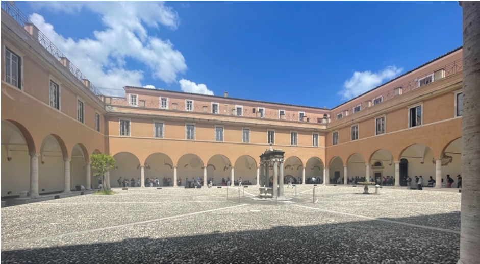
Courtyard of the Formal Structures for Computation and Deduction conference venue, in the building of Civil and Industrial Engineering on the campus of Sapienza University of Rome.
