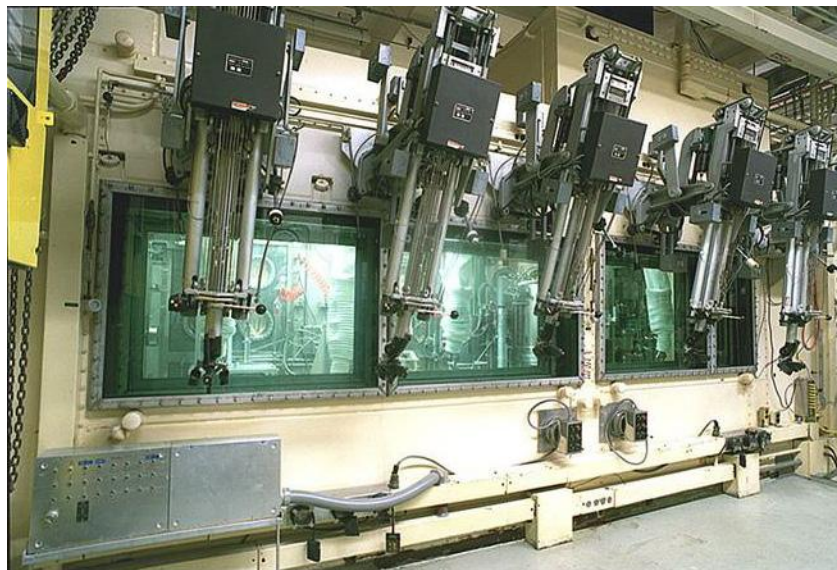
FIGURE 3-24 | IAAC AT INL'S SPACE AND SECURITY POWER SYSTEMS FACILITY
