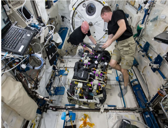
Carbon Dioxide Removal Assembly (CDRA) Maintenance. Photo: NASA (2015)
