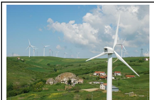
Following an SBIR contract to develop wind power technology suitable for Mars, more than 200 NASA-derived Northern Power 100 wind turbines are in operation across the world. The turbines shown in this picture are from an installation in the Italian countryside.
