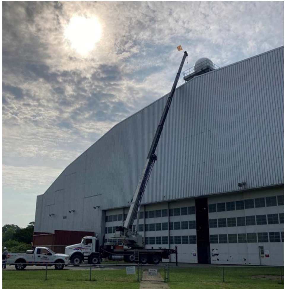
The LSTAR-2 being lifted into the radome.
