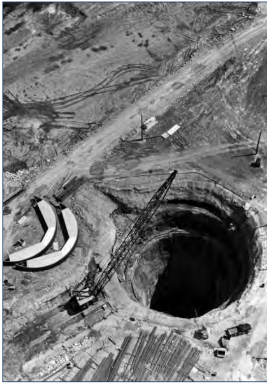
Construction of the B-2 site required the excavation of a 180-foot-deep hole, pictured here in 1965. (Source: Glenn Research Center, file photo number 01264)
