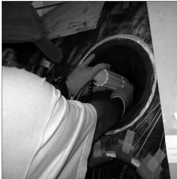
Quality assurance inspector James Allen Atwell is using the RCS fuel hole inspection device to look into a nozzle in bay 2 of the Orbiter Processing Facility.
