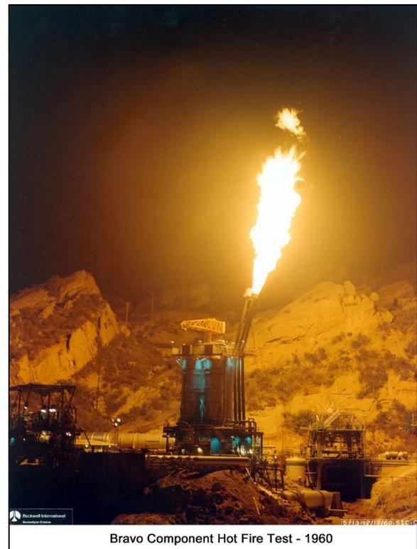
Figure 5-11. 1960 Photo of Bravo Test Stand undergoing a hot fire test.
