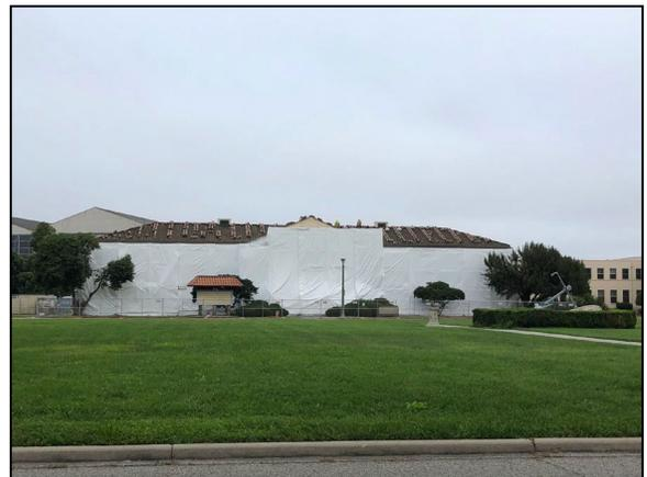
Figure 4-6. Exterior asbestos containment at Building 25.
