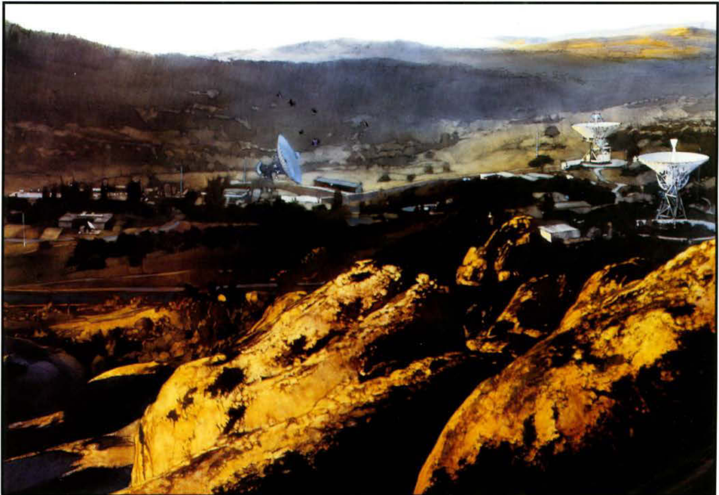
Madrid Deep Space Communications Complex
