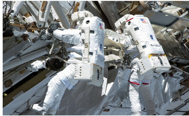
NASA astronauts during a May 2013 leak repair spacewalk.
