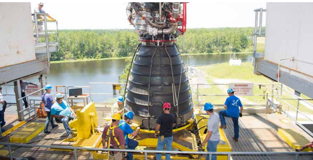
Right: Technicians ready a developmental RS-25 engine number 0525 for installation on the A-1 test stand at Stennis Space Center on July 23 in preparation for a series of hot-fire tests. Once unloaded from the delivery platform, the engine will be lifted by crane into its test position. NASA conducted the series of hot-fire tests in mid-August. Image credit: NASA
