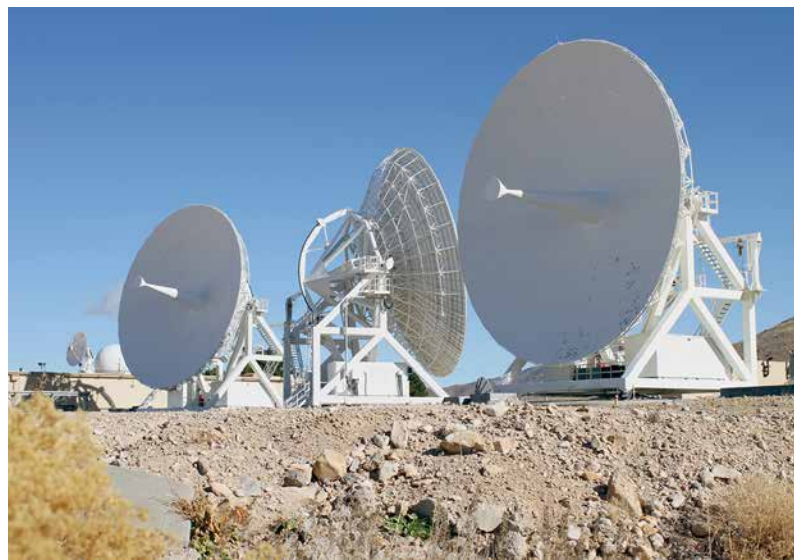
Above: The White Sands Ground Terminal in Las Cruces, New Mexico, comprises several antennas that provide communications to spacecraft as part of NASA’s Space Network. Image credit: NASA/Amber Jacobson
