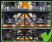
FIRST INTEGRATED POWER UP
