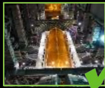
START INSTALL OF INTERNAL PLATFORMS
