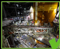
UMBILICAL CONNECTS COMPLETE
