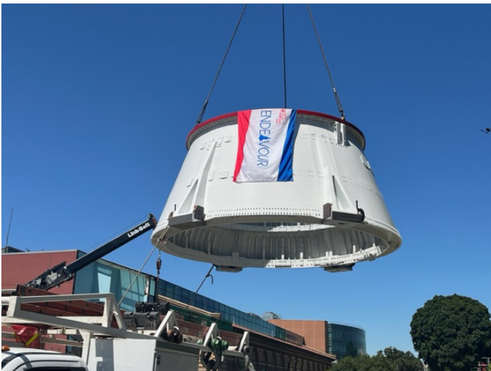
Photo of an aft skirt being lifted into the new building.
