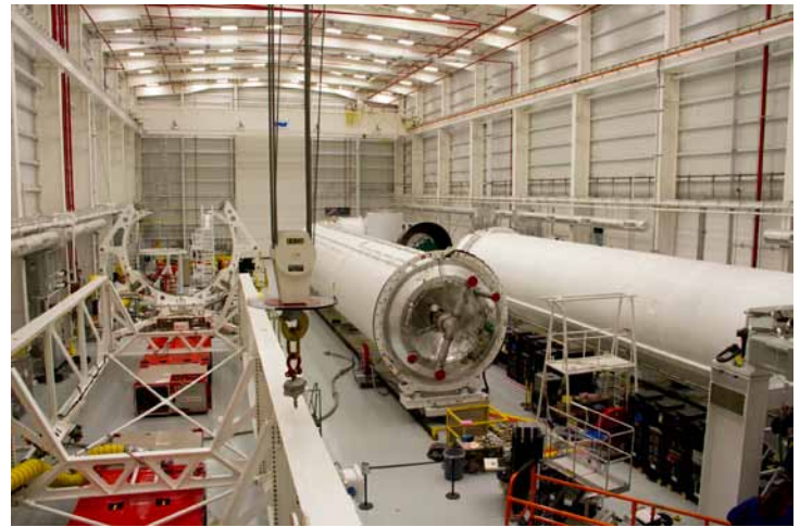
Figure 3-13. Horizontal Integration Facility
