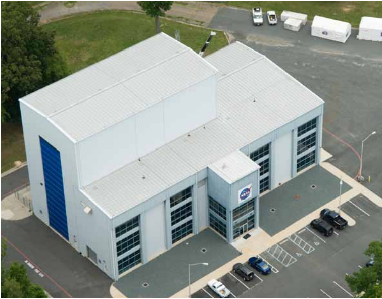
Figure 3-10. H-100 Payload Processing Facility (PPF)
