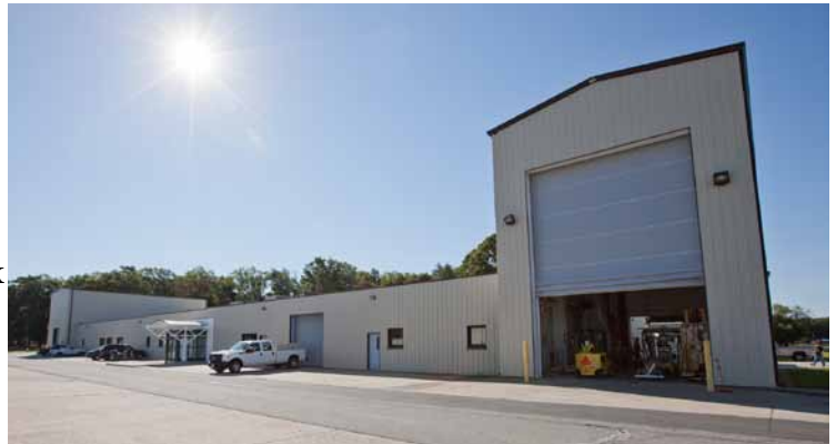
Figure 3-15. Multi-Payload Processing Facility (MPPF)
