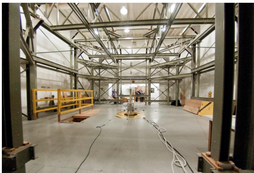
Figure 6.2.8-1 The Magnetic Test Facility at Wallops
