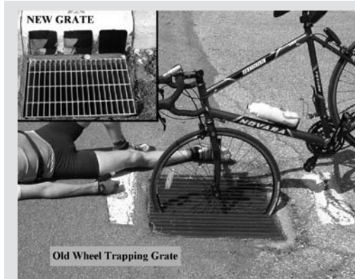
The replaced bike grate at the center improves safety for bike riders at Ames.
