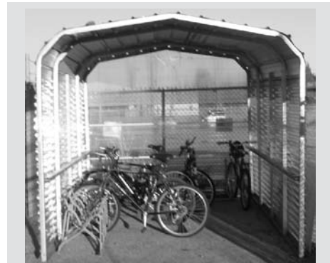
The newly installed bike shelter at Ames located just inside the Ellis gate.
