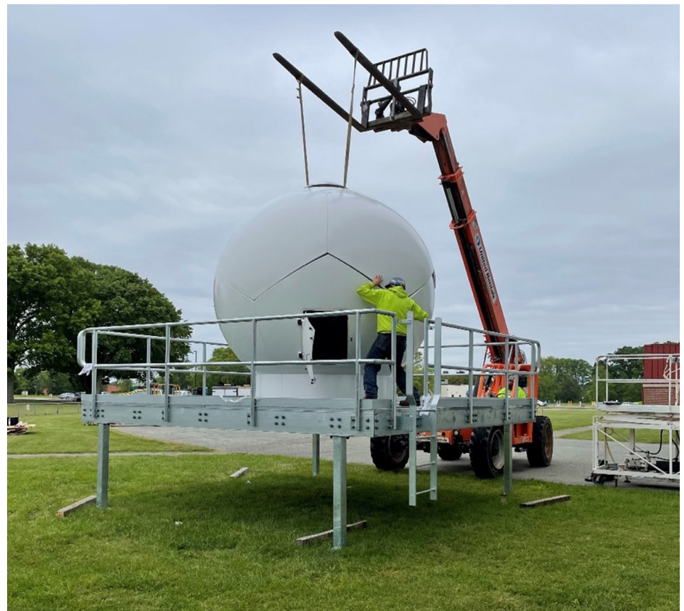
Installation of the Radome on the Radar Platform.
