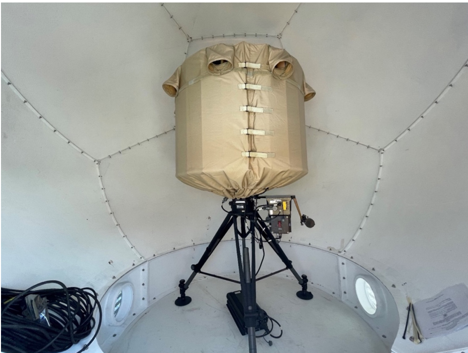
LSTAR successfully assembled inside the newly installed radome.
