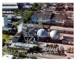
Figure 4.1.0.1. NASA Ames Research Center Arc Jet Complex
