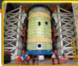
SLS Intertank Test Fixture (2.5 million lb of steel)
