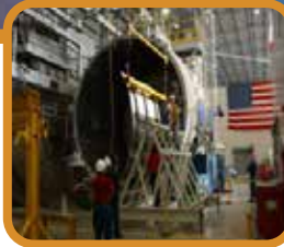
Shroud Installation in V20
