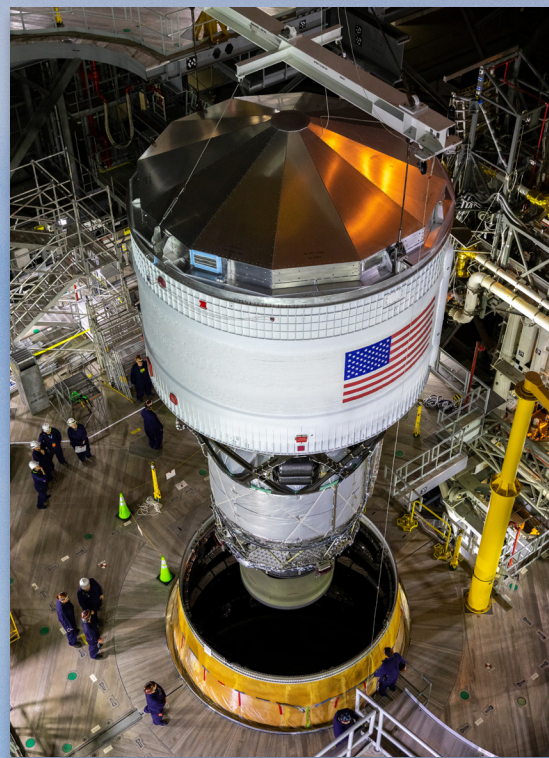
Above: ICPS mating with SLS core stage. Right: Multiple interfaces exist between the ML and the Artemis I vehicle. The crew access arm and Orion service module umbilical are located at 280 feet, the ICPS umbilical complex is next at 240 feet, followed by the vehicle stabilizer system and the core stage forward skirt umbilical at 200 and 180 feet, respectively.
