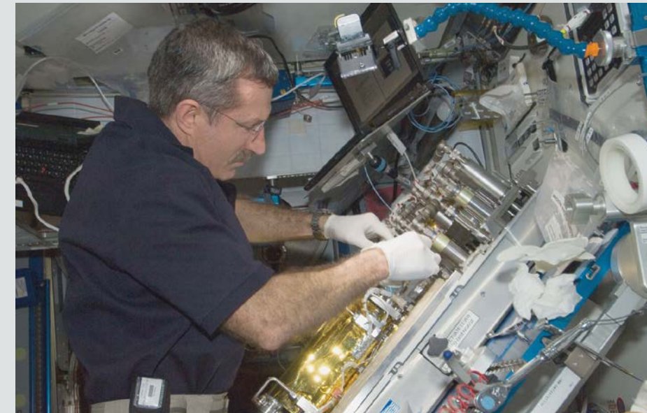
At a workstation in the ISS Harmony node, astronaut Dan Burbank replaces a catalytic reactor in the water recovery system.
