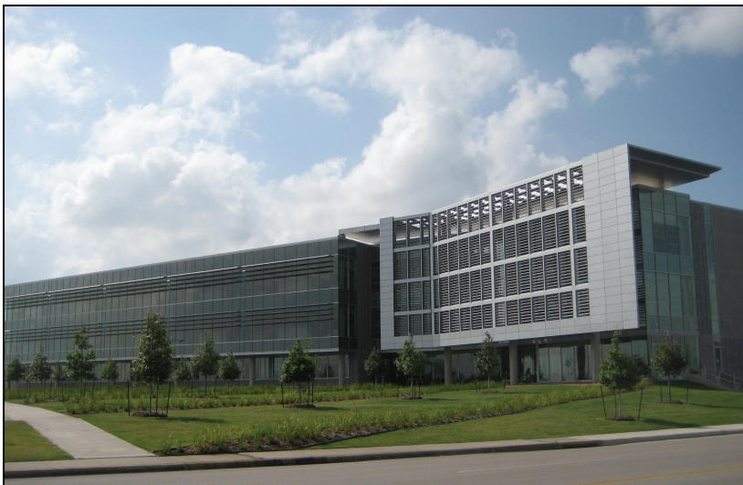
Figure 1 - Building 20, Johnson Space Center, Houston, Texas
