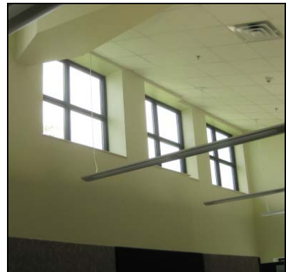
Figure 17 - Clerestory Windows, Building 265, Johnson Space Center
