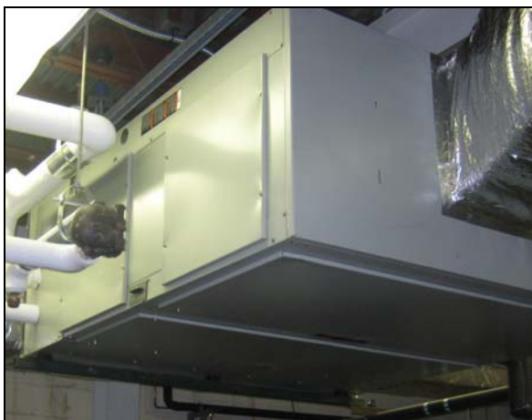
Figure 3 - Building 1221B, Langley Research Center
