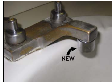
Figure 6 - Example Faucet and Aerator Building 1267A, Langley Research Center
