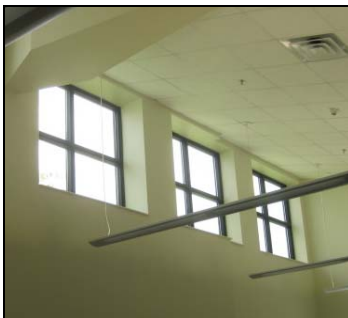
Figure 6 - Clerestory Windows, Building 265, Johnson Space Center
