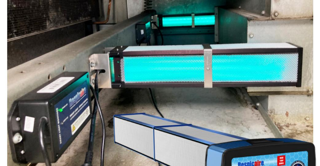
Two OXY 4-MB air purifiers from Respicaire are installed in the air handling unit at Synergy Flavors Inc. in Wauconda, Illinois. Credit: Jensen's Plumbing & Heating
