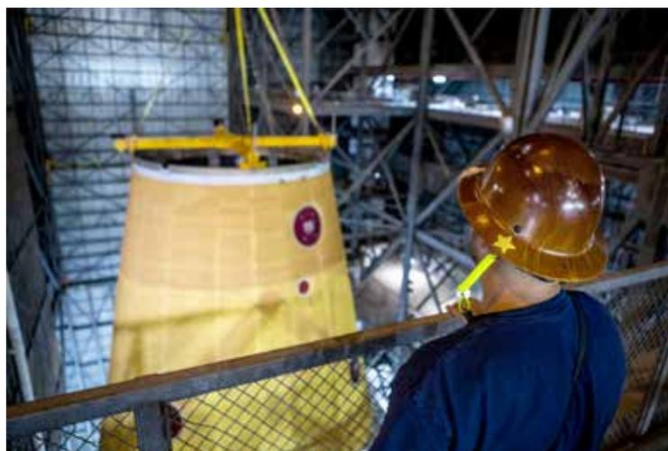
The LVSA for the Artemis I SLS is moved into position on the core stage at the Vehicle Assembly Building (VAB).
