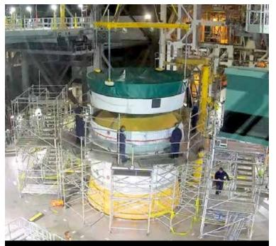
The Artemis I Orion stage adapter (OSA) is stacked on top of the ICPS.
