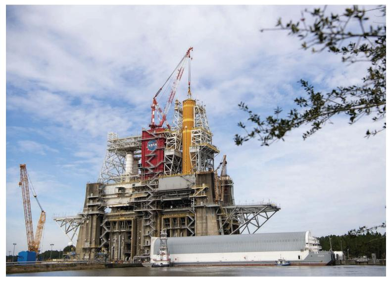
The core stage that will fly on the Artemis I mission is installed in the B-2 Test Stand at Stennis Space Center near Bay St. Louis, Mississippi, for Green Run testing. The test series is scheduled to take place over several months.
