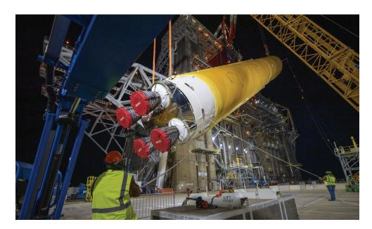
Crews used large cranes to lift the Artemis I core stage for installation in the B-2 test stand. The stage includes the liquid hydrogen and liquid oxygen tanks, four RS-25 engines and the vehicle's avionics and flight computers. When it is filled with all 733,000 gallons of propellant for flight, the stage will weigh more than 2 million pounds and will have the power to reach Mach 23 – faster than 17,000 miles per hour.
