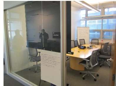
Figure 49 – Interior Wall Glazing
