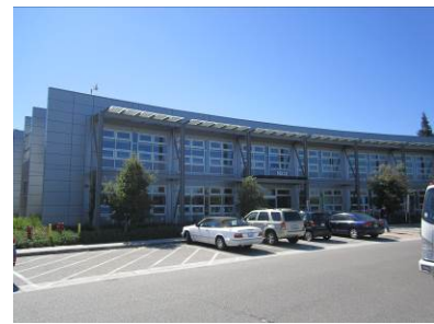
Figure 13 – Exterior View of Facility
