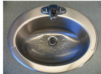
Figure 29 – Hand-Sensing Low Flow Faucet
