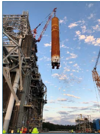
SLS Core Stage removal from SSC B2 Test Stand
