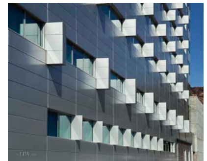
Exterior window shading provides both function and a distinctive design feature.
