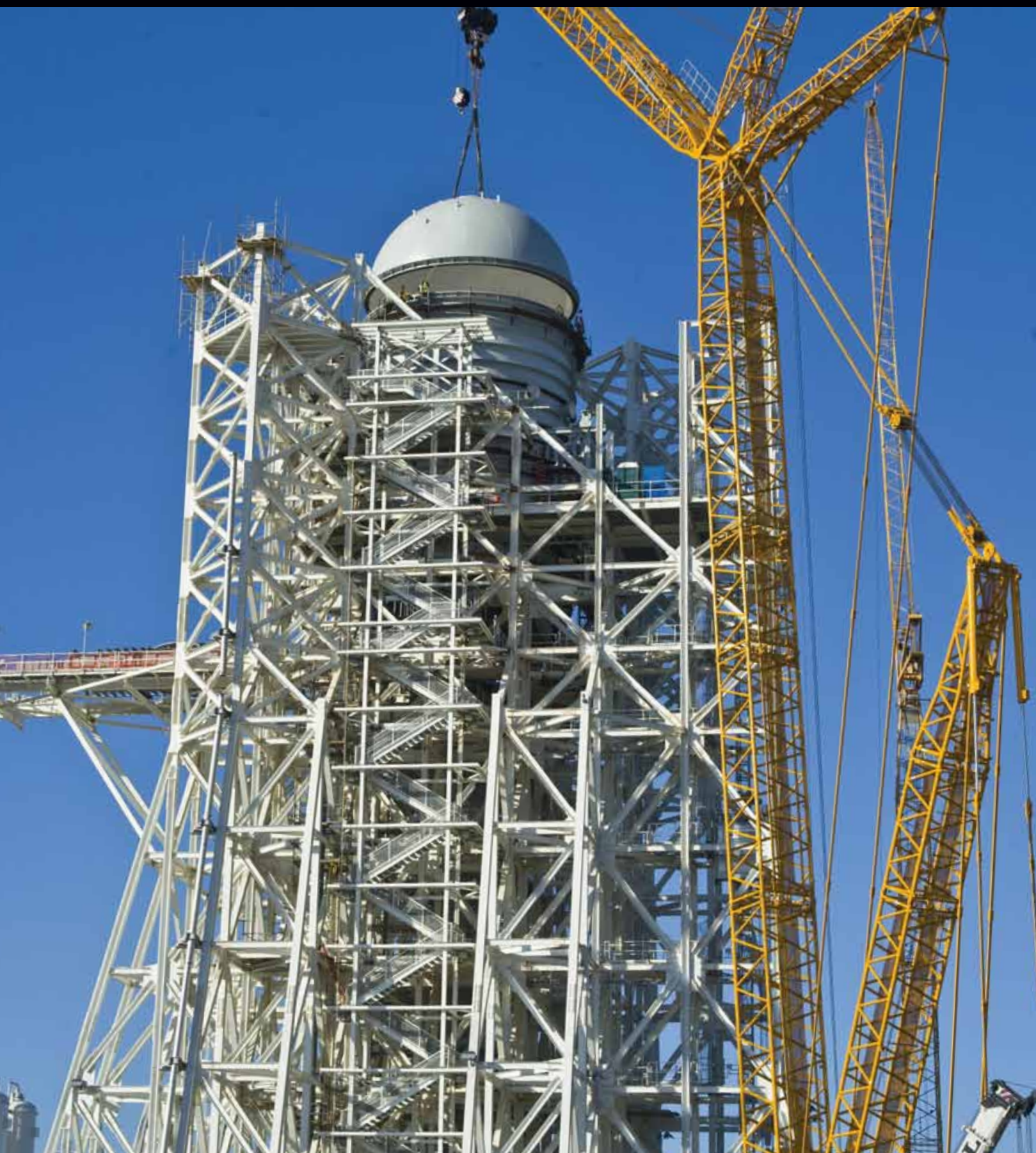
The A-3 test stand under construction at SSC
