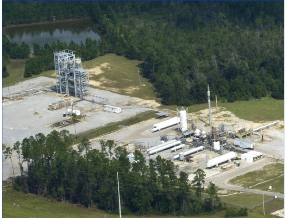
An aerial photo shows Cell 1 (l) and Cell 2 (r) of the E-2 Test Facility (formerly known as the High Heat Flux Facility) at Stennis Space Center. Since its construction in the 1990s, Cell 1 has been modified to support advanced component and engine development projects. Its capabilities include supporting up to 100,000 pounds of thrust from combustion devices or turbopumps with liquid oxygen, liquid nitrogen, liquid hydrogen, isopropyl alcohol, refined petroleum, water, gaseous hydrogen, gaseous oxygen, gaseous methane, and gaseous nitrogen. Photo credit: (NASA/SSC)
