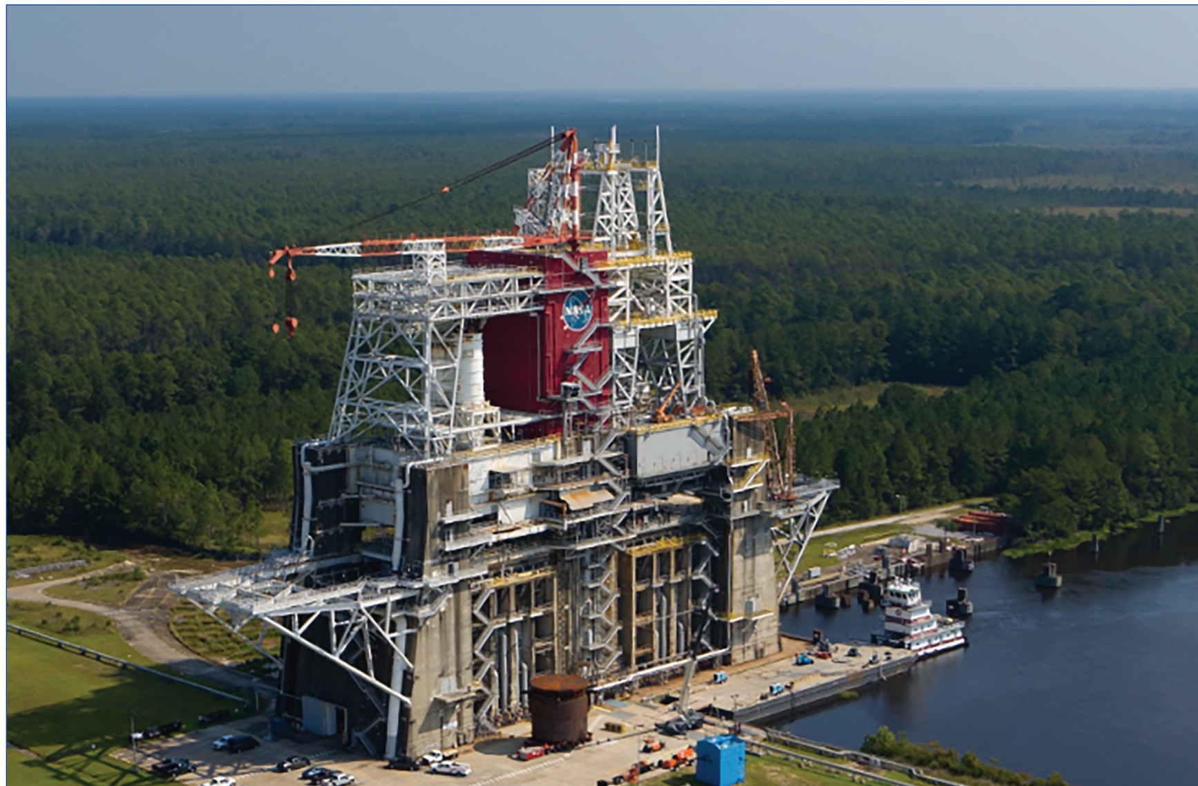
(Above photo) A drone photo shows the interstage simulator component sitting on the tarmac of the B-2 Test Stand at NASA's Stennis Space Center on Sept. 21, 2022. In upcoming months, Stennis will prepare the unit to be installed on the stand to support testing of the Exploration Upper Stage
