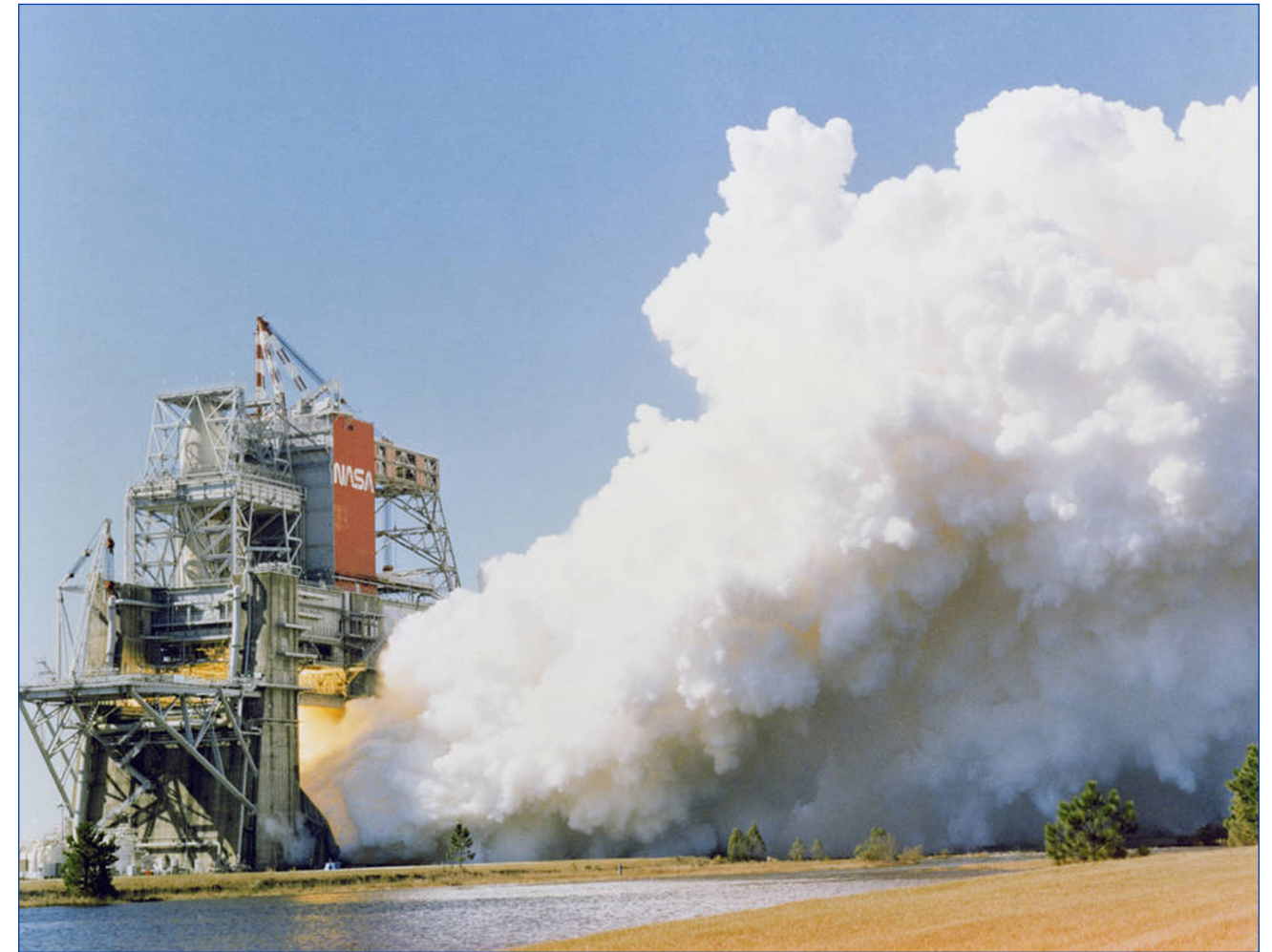
(Top photo) A Dec. 17, 1979 photo shows a hot fire test of the main propulsion test article (MPTA) on the B-2 Test Stand at NASA's Stennis Space Center, then known as National Space Technology Laboratories. MPTA testing involved installing a shuttle fuel tank, a mockup of the shuttle orbiter, and the vehicle's three-engine configuration on the stand, then firing all three engines simultaneously, as would be done during an actual launch.
