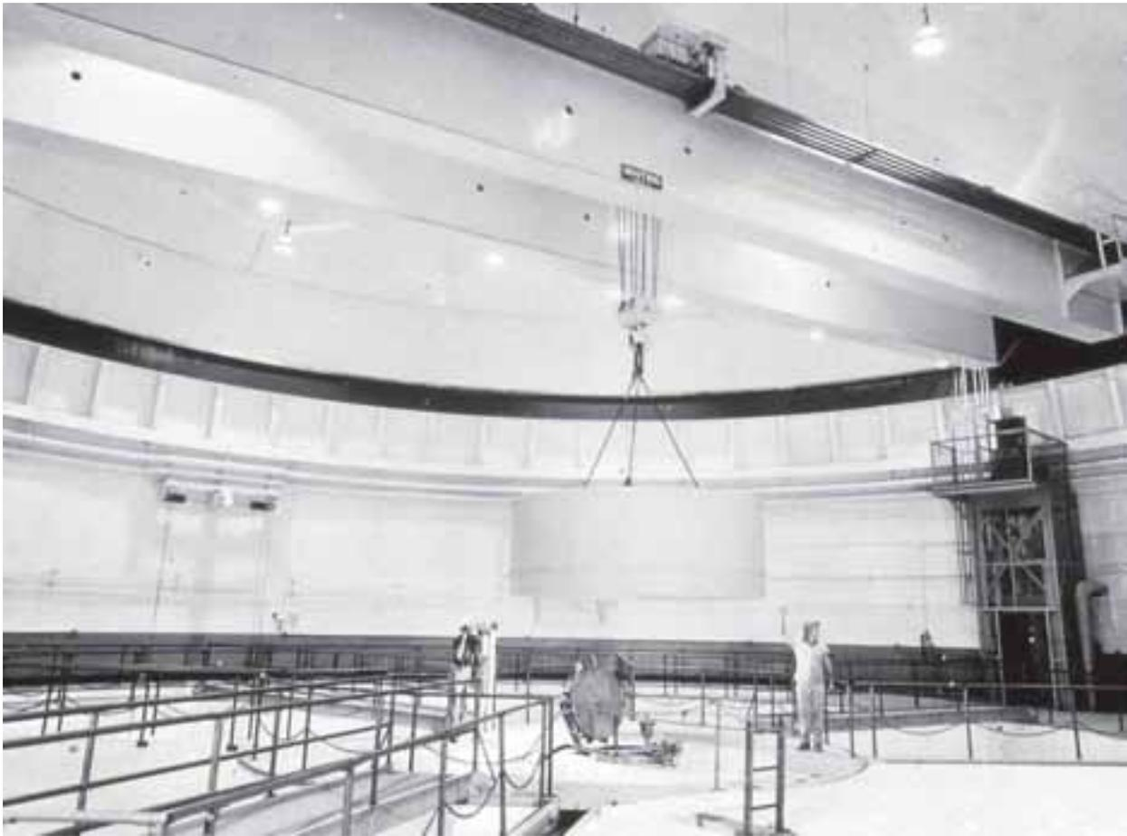
*Image 64: Two men standing on the lily pad guide a crane to remove the third of three large, white, twenty-ton shrapnel shields that nest over the pressure tank. The shields were then stacked off to the side until it was time to reposition them on top of the pressure tank. Since the support beams could rotate 365 degrees, the overhead crane could reach any location in the containment vessel. The pressure tank hatch is open. (1959) (NASA CS-18228)*
