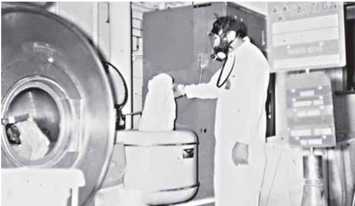
*Image 82: A Plum Brook technician wearing protective clothing and a mask washes contaminated clothing. The clothing was worn again after it was decontaminated and laundered. The wash water had to be treated as radioactive waste. (2001) (NASA C-2003-841)*
