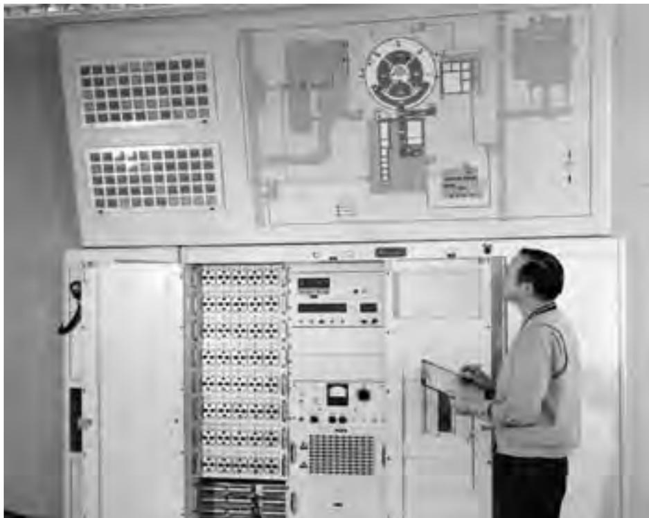
Tom Junod, the Health and Safety Officer, looks at radiation sensing monitoring equipment. The color of the lights indicated the presence or absence of radiation. (NASA 1961\_55636)
