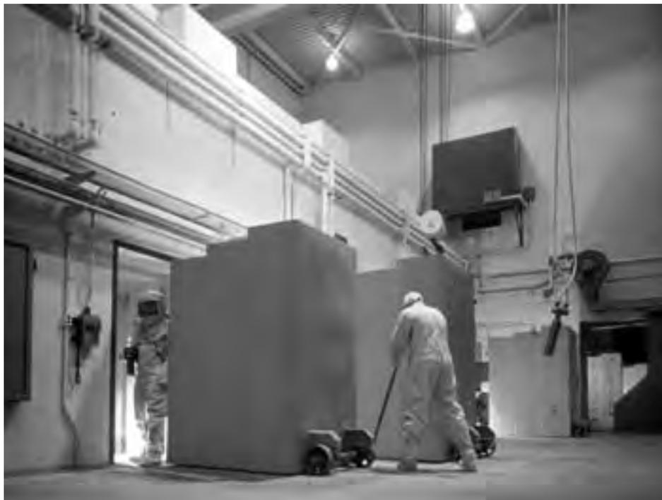
*A technician emerges from the rear of the hot laboratory in full protective clothing. Another technician wheels open the massive 63-inch-thick concrete door plug. (NASA CS-22203)*
