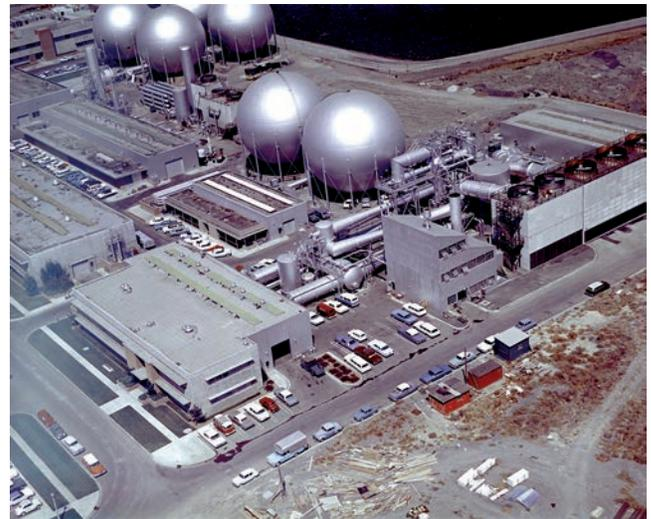
While the HFF generated an enthalpy of 30,000 Btu per pound, the peak heating lasted mere milliseconds. These tunnels worked well for studying reentry aerodynamics, but the heating time was of little use for testing ablative materials. Ablative materials include ceramics, quartz, teflon, or graphite composites that slowly melted
