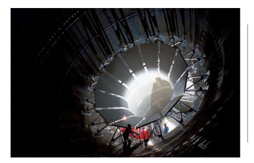
Diffuser and contraction vanes during 1996 upgrades to the Unitary plan wind tunnels.
