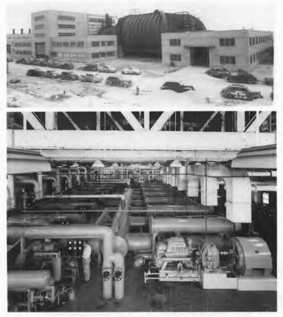
Top: The Altitude Wind Tunnel urgently needed for full-scale engine testing. Bottom: Innovative Carrier compressors chill the tunnel's airstream.
