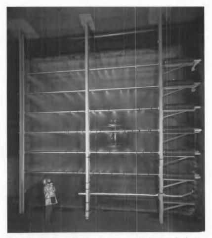
Vernon Gray investigates the new spray system, completed in 1950, for the Icing Research Tunnel.
