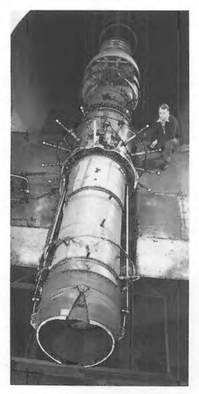
A Westinghouse axial-flow turbojet fitted with NACA variable area nozzle for afterburner studies in the Altitude Wind Tunnel, 1951.
