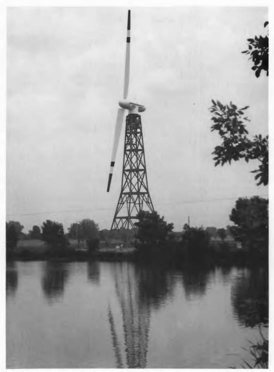
100-kilowatt wind turbine at Plum Brook.
