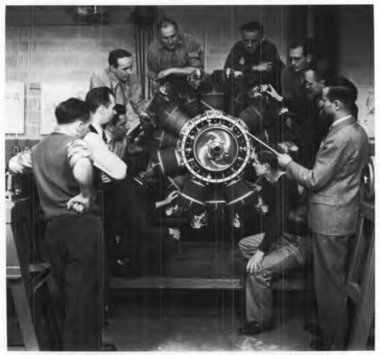
A representative from Wright Aeronautical instructs staff on the principles of the radial engine.
